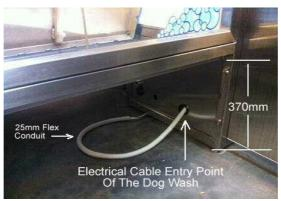
The above picture shows the main electrical cable entry point into the dog wash. Once you have run the cable and conduit to this point, leave another 900mm for the termination inside the cabinet.
