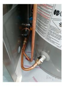
Shown picture below shows the water entry point for a K9000 2.0 with a hot water storage service.
