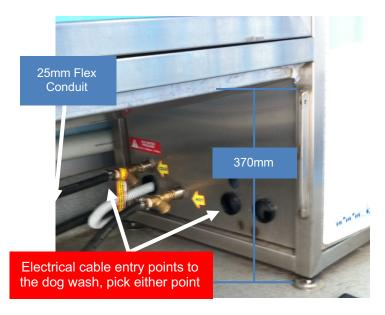
The External Hot Water Unit will need to be wired into the gland by an electrician following the Hot Water Unit's installation process.
